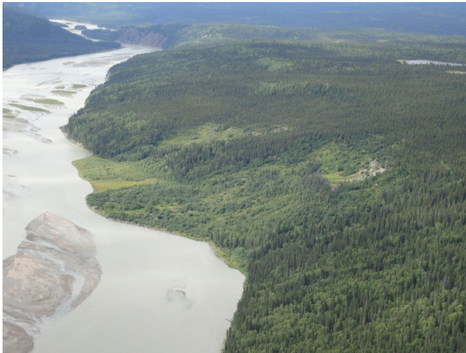
Figure 9. Rotational Slide, Earth Slump, North Abutment, near RM 198, Upstream of Confluence with Watana Creek (Sheet 12-7).
