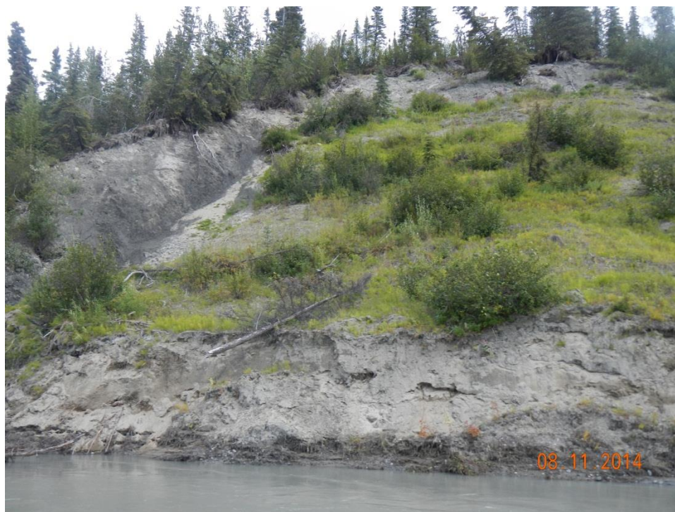
Figure A.2-17- Active landslide in till near PRM 251.8 (P400).
