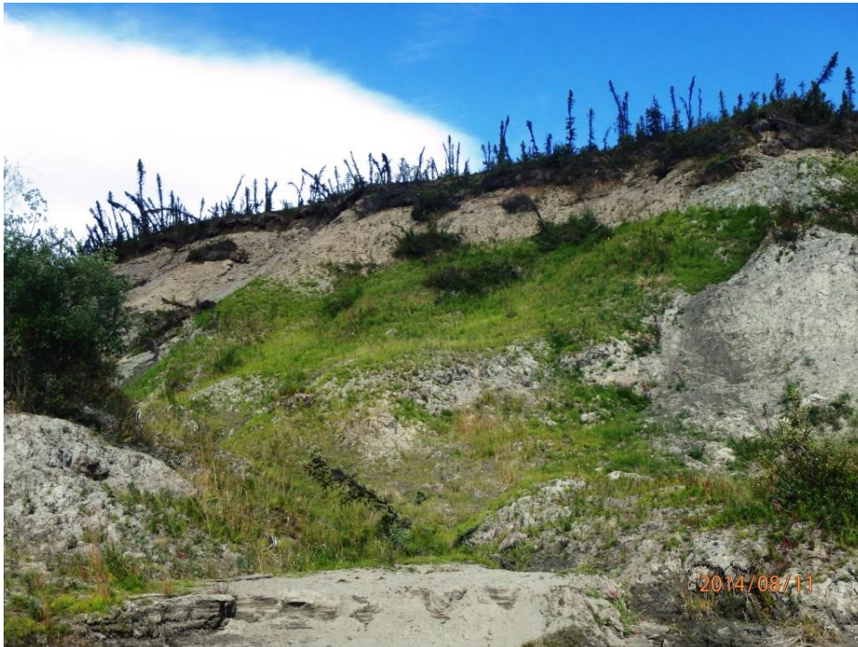
Figure A.2-24 – Vegetation unable to establish on very actively eroding unstable bank face (P903).
