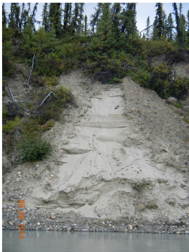
Figure A.1-15 – Active landslide near PRM 274.8 – sands and fine gravel in glacio-deltaic deposits (P956).
