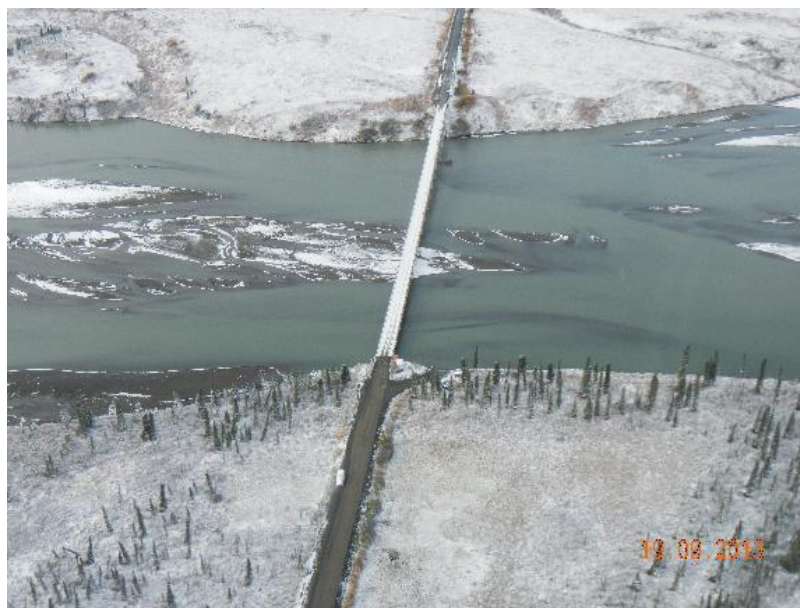
Figure A.1-2 – View east of Denali Highway Bridge at PRM 292. Susitna River, flow from right to left (P5582).
