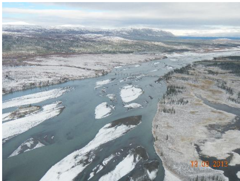
Figure A.1-1 – View upstream towards Denali Highway Bridge at PRM 292 (P5580) 1 .
