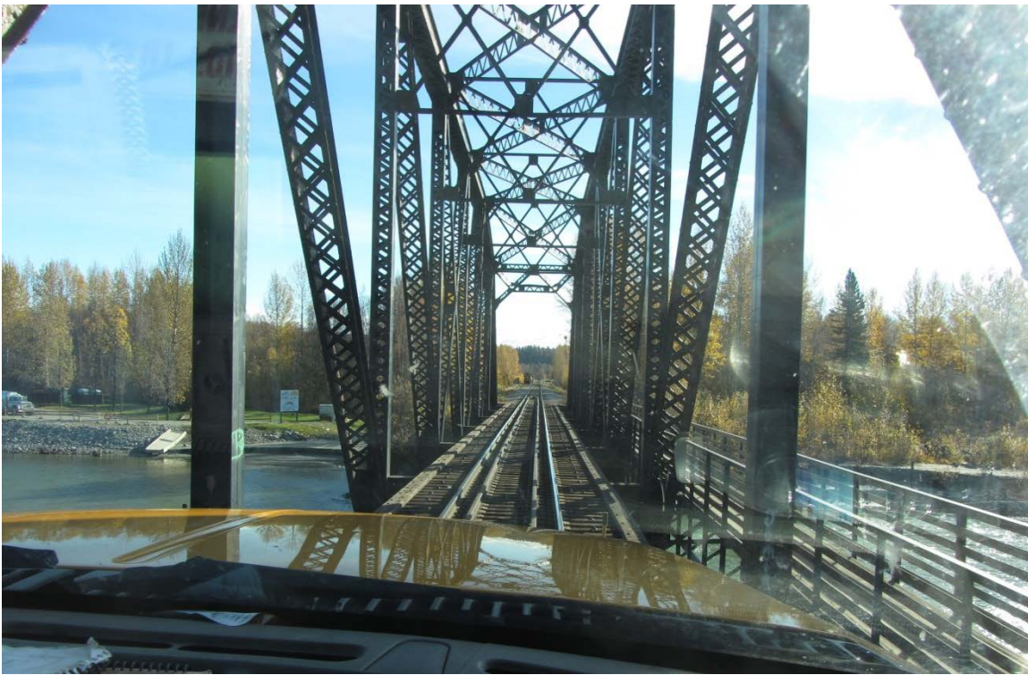
Figure 13.3-13. Talkeetna River Bridge
