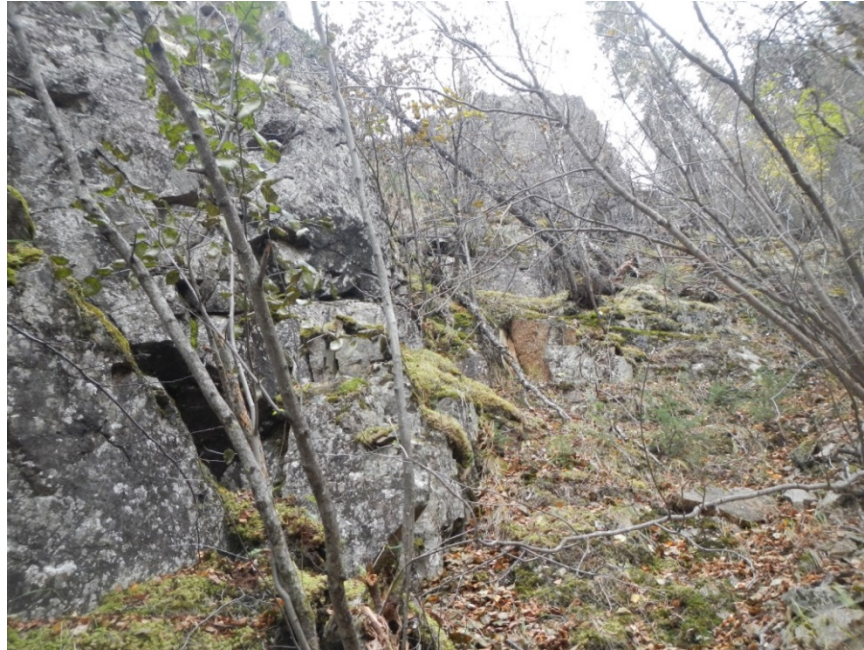
Figure 6.3-23. 75 ft. High Cliff on Right Abutment Forming the Downstream (Southwest) Boundary of GF5
