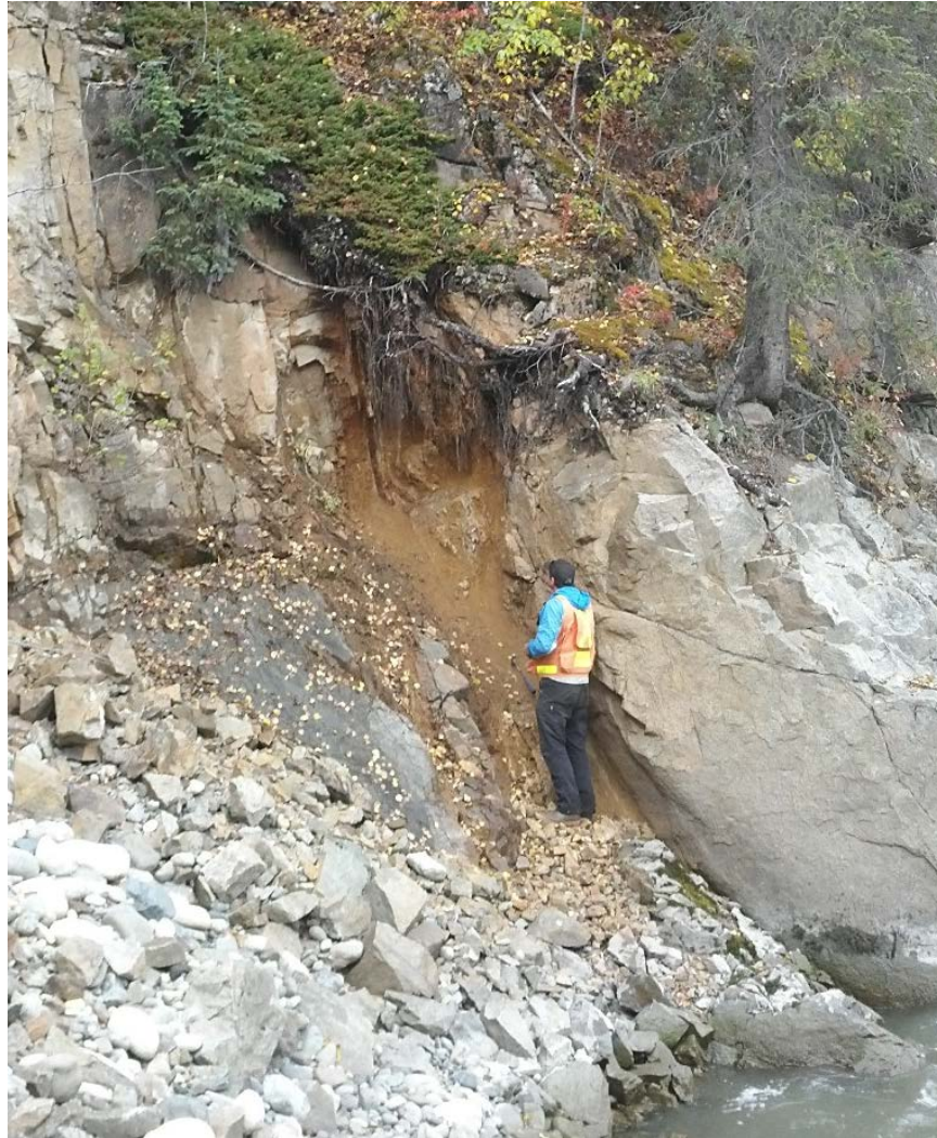
Figure 6.3-18. Shear Zone in Outcrop at GF1.
