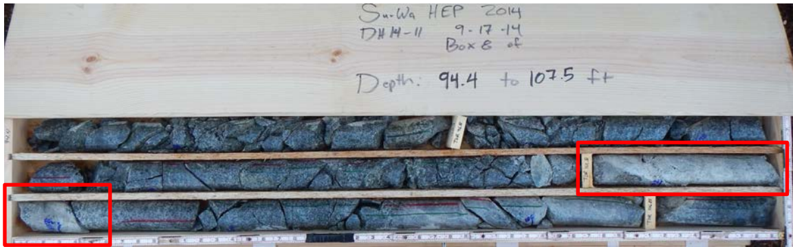
Figure 6.3-24. Rock Core from DH14-11 with Closely Fractured Rock and Shear Zone at Depth of about 102 ft. (red box)
