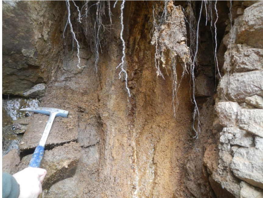
Figure 6.3-19. Close-up of 3 to 4 ft. Wide Shear Zone at GF1
