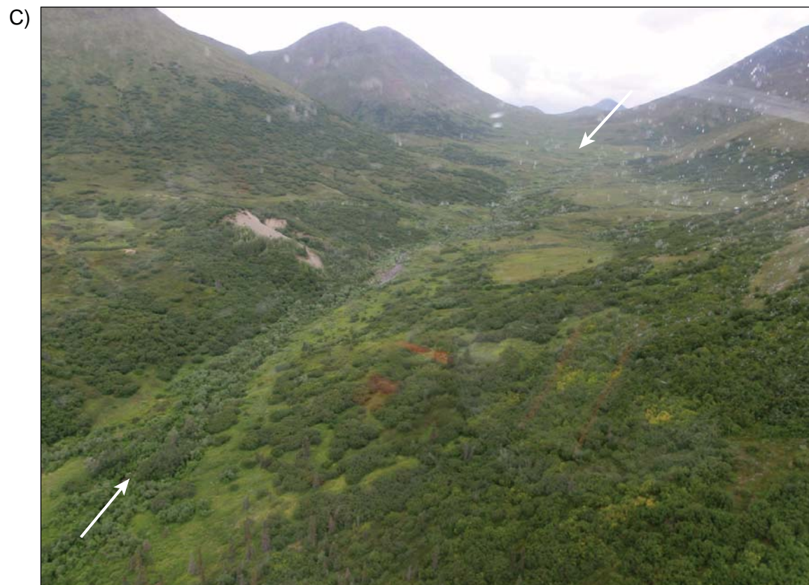
View looking up-valley at incised drainage that coincides with mapped lineament and previously mapped fault.
