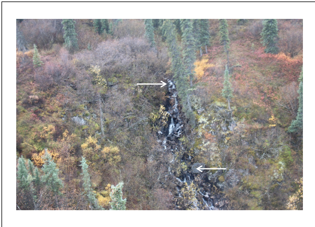
Figure A1. Barrier A in Unnamed Tributary 189.7. Fixed seasonal boulder cascade, 29 ft in height and horizontal length of 36 ft with an average channel gradient of 82 percent.
