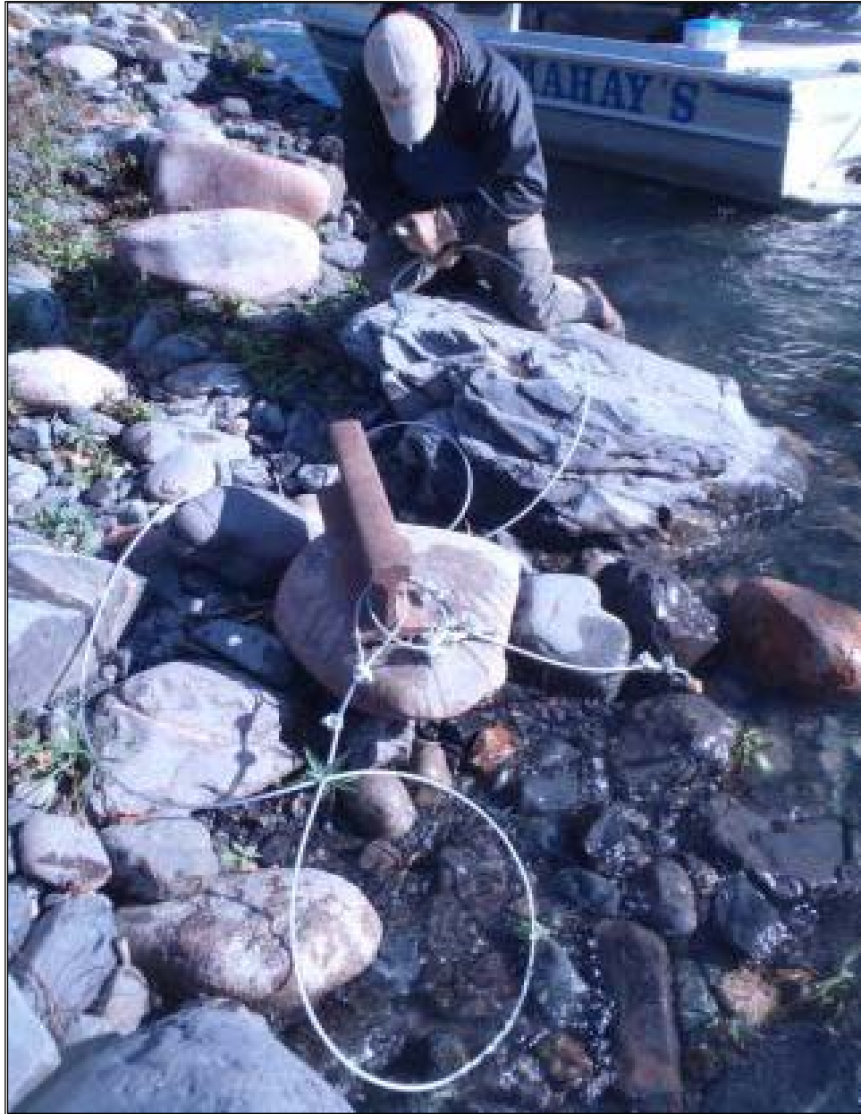
Photo A-28b. Buoy installation at PRM 152.3 – Portage Creek
