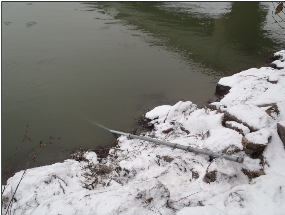
Photo A-7c. Pipe Installation at PRM 87.8 – Susitna at Parks Highway East
