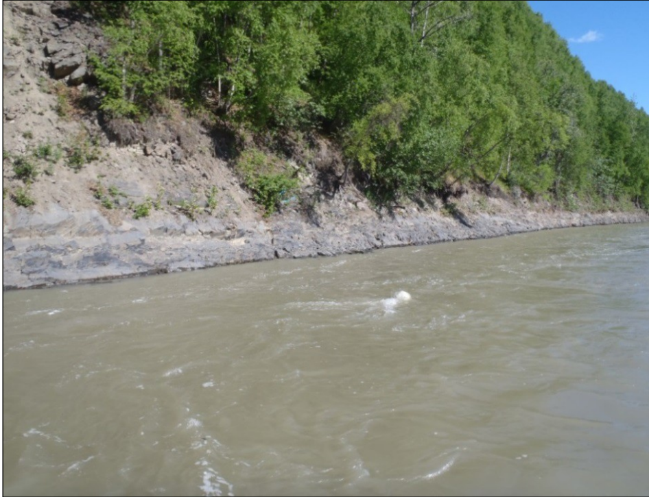
Photo A-14b. Buoy system installed at PRM 124.2 – Up-River of Curry Fishwheel Camp
