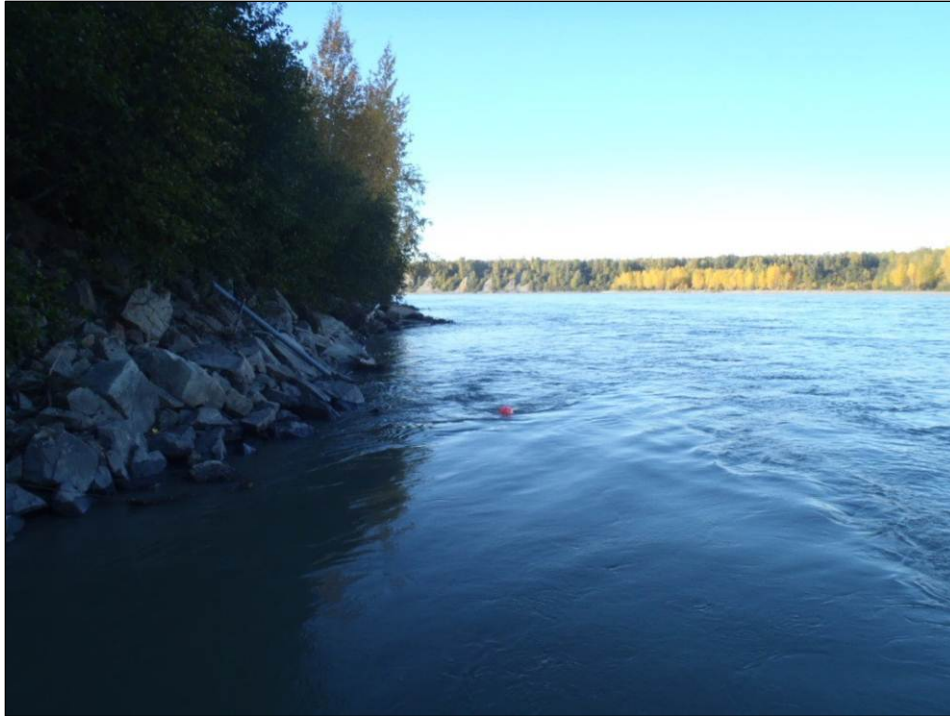
Photo A-7b. Buoy and pipe Installations at PRM 87.8 – Susitna at Parks Highway East
