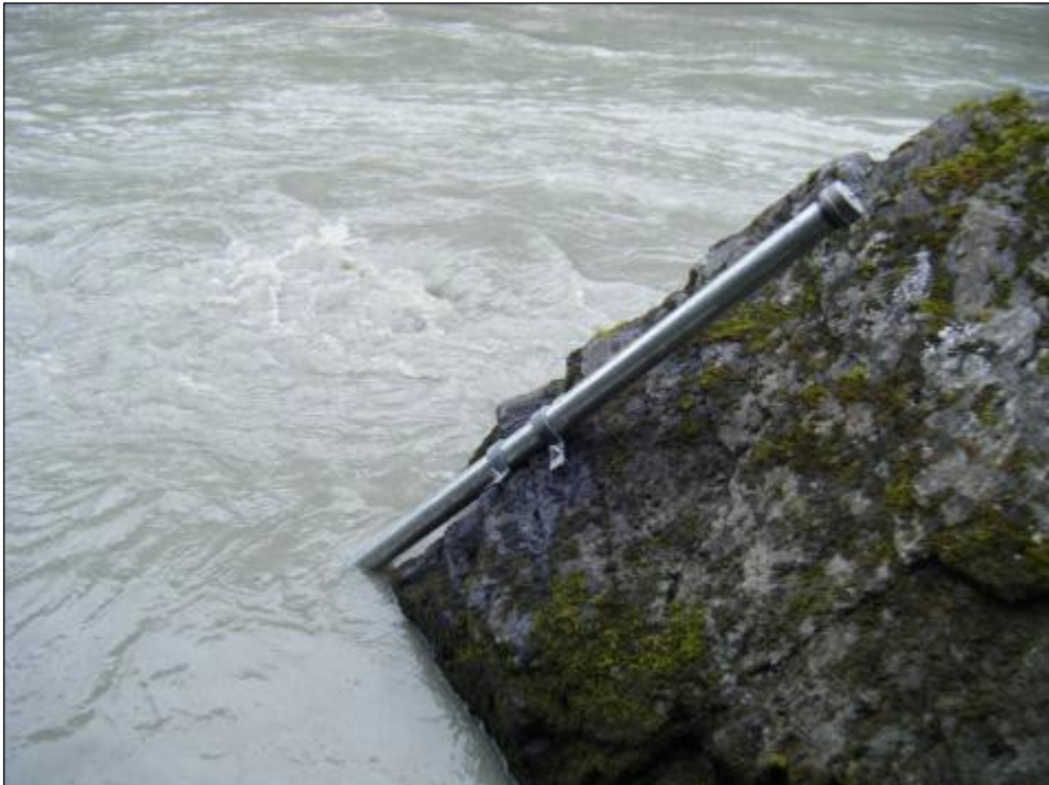
Photo A-29c. Pipe installation at PRM 152.7 – Above Portage Creek
