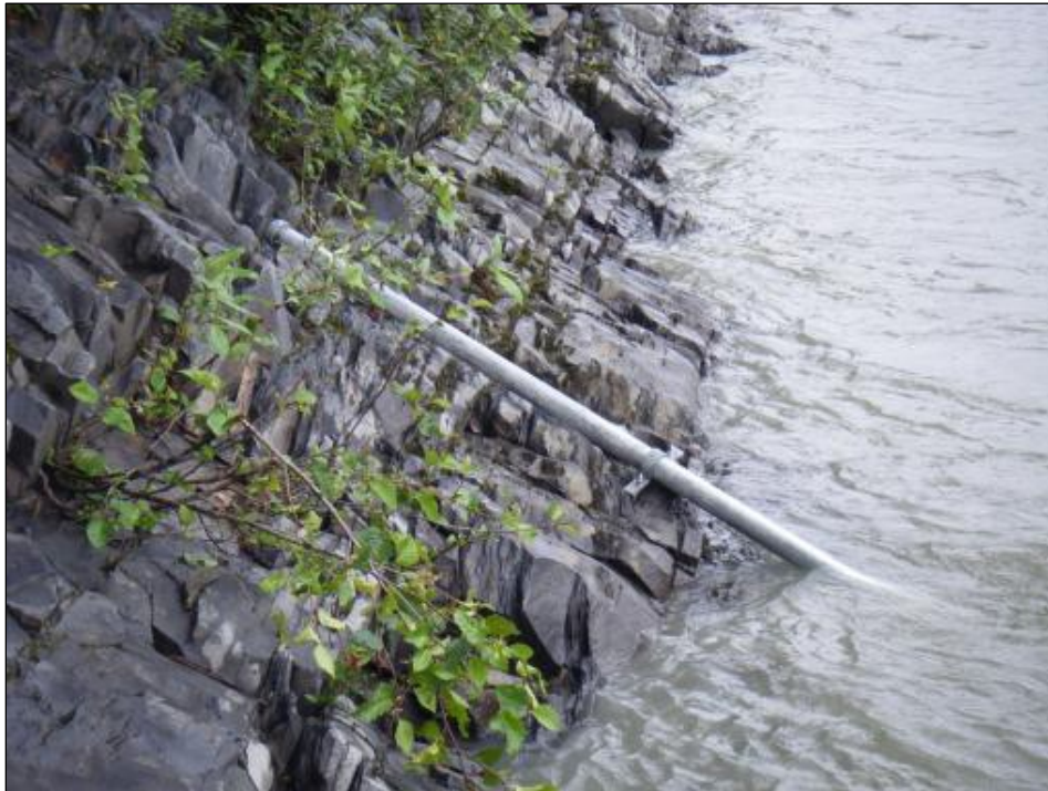
Photo A14-c. PRM 124.2 – Pipe system at Curry Fishwheel Camp
