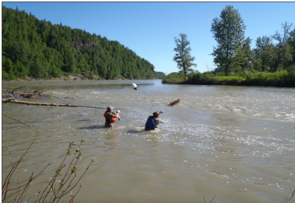
Photo A-15c. Installing buoy system at PRM 129.6 – Slough 8A
