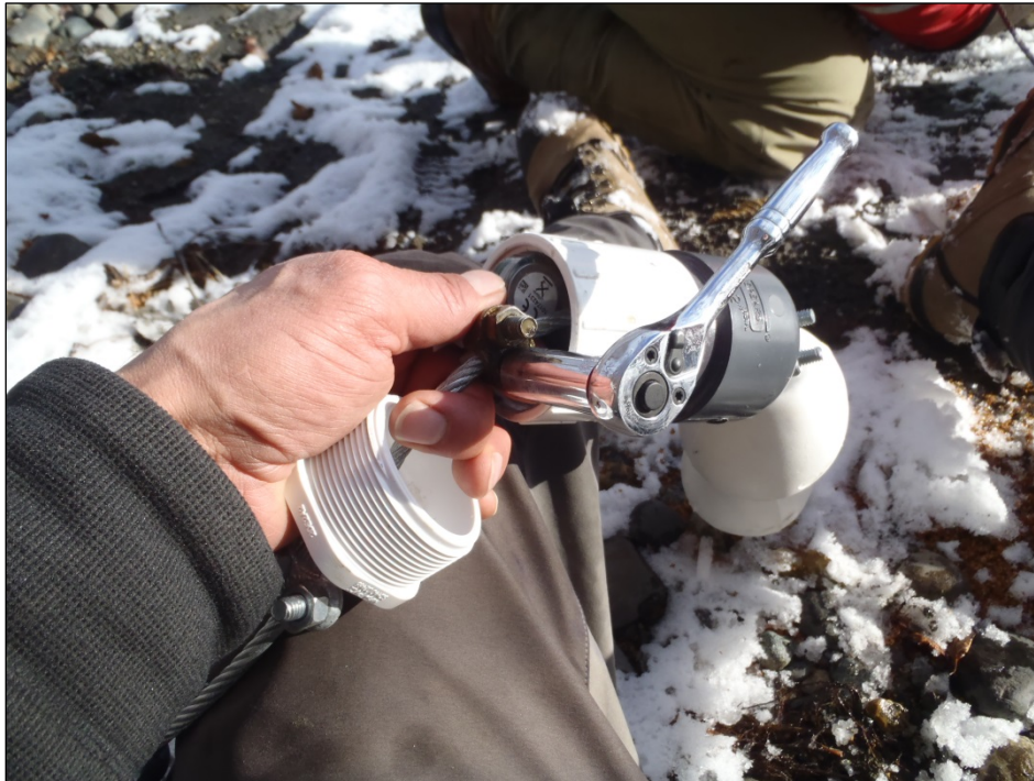
Photo A-30c. Installing thermistor in overwinter system.
