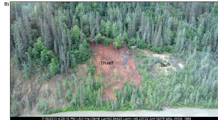
View looking east along lower river bank at apparent alternation zone distinguished by color contrast, possible juxtaposition of Triassic metabasalts and undifferentiated Tertiary sediments. This location is east of the mapped projections of the Talkeetna fault.
