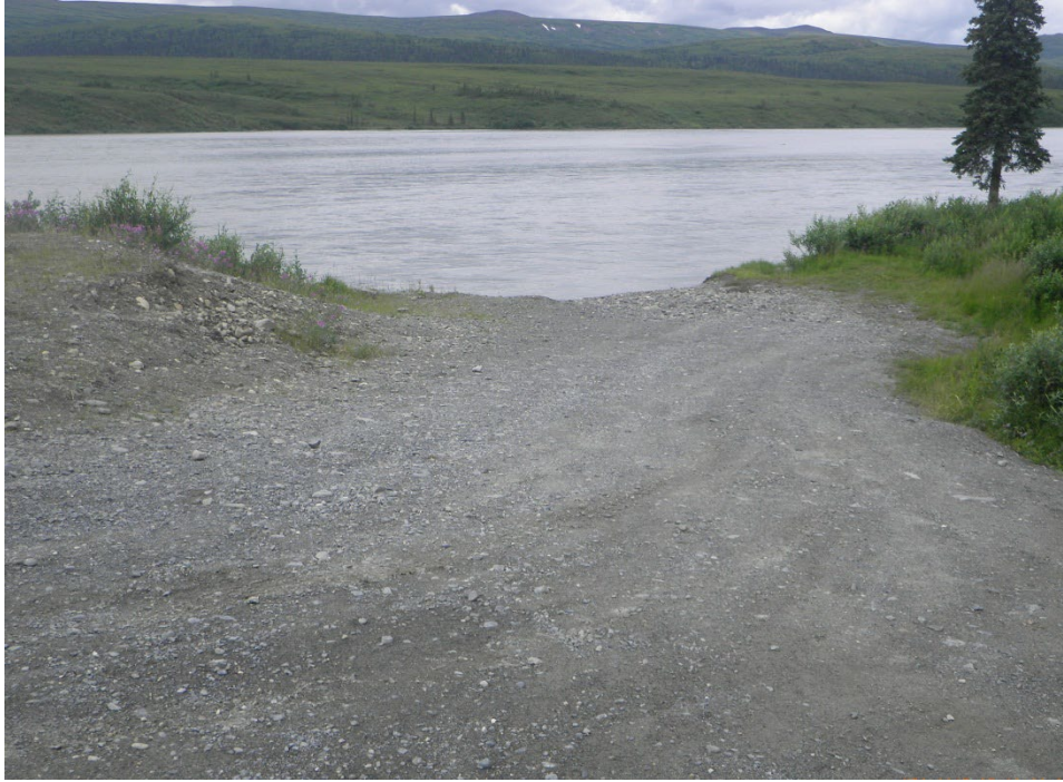
Photograph K-9. Susitna River Access Point at Denali Highway Bridge
