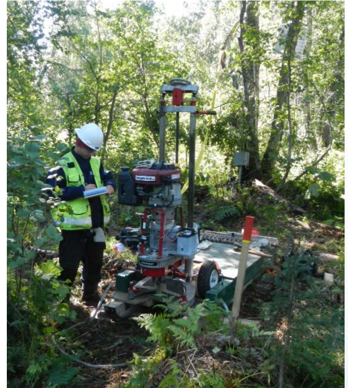
Getting ready to drill next well location in FA104 – Whiskers Slough, Riparian data station location in forest, August 25, 2013
