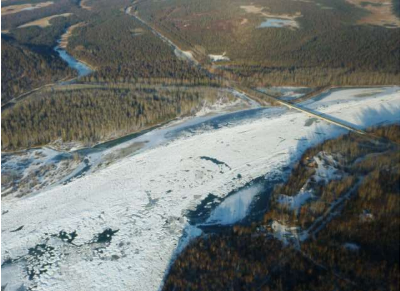
Figure 5.6-7. Parks Highway Bridge at RM 84 on November 7, 2012, after ice cover progression. Note flooded gravel bars on both sides of the river.
