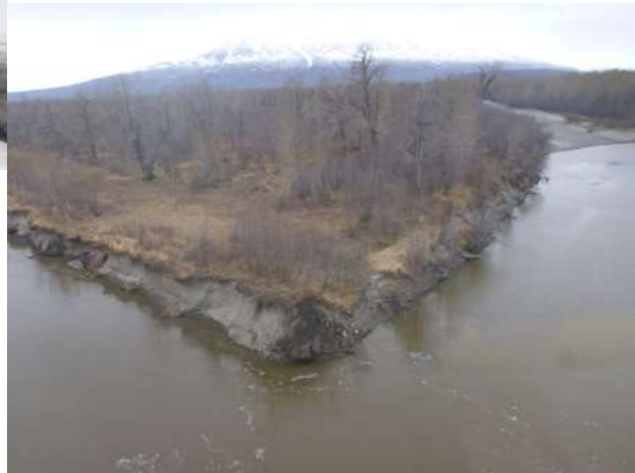
RM 10, PRM 15 eroded bank, May 10, 2012
