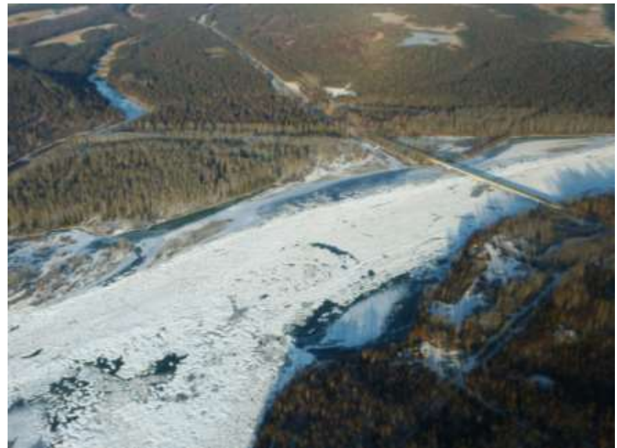
Parks Highway Bridge, November 7 th
