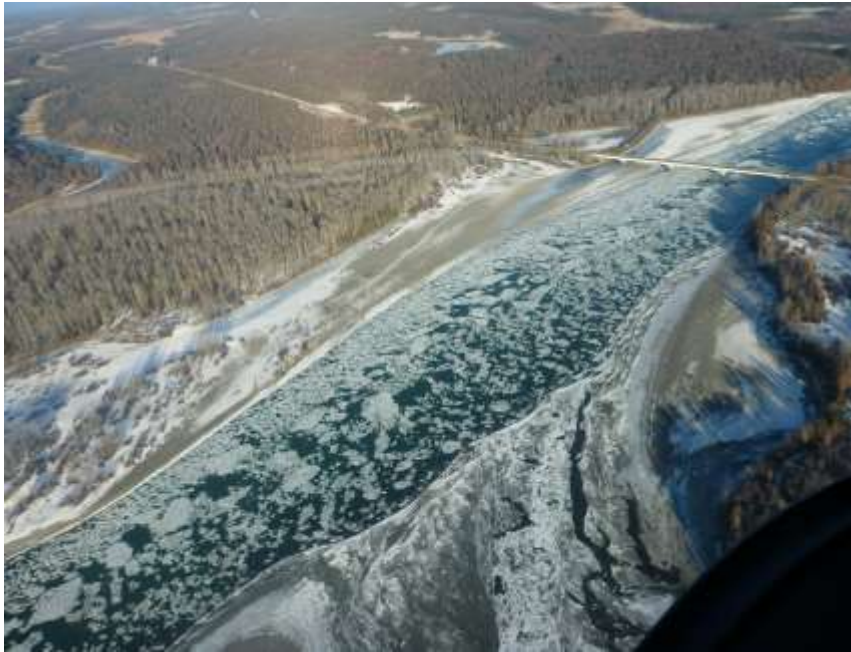
Parks Highway Bridge, November 1 st
