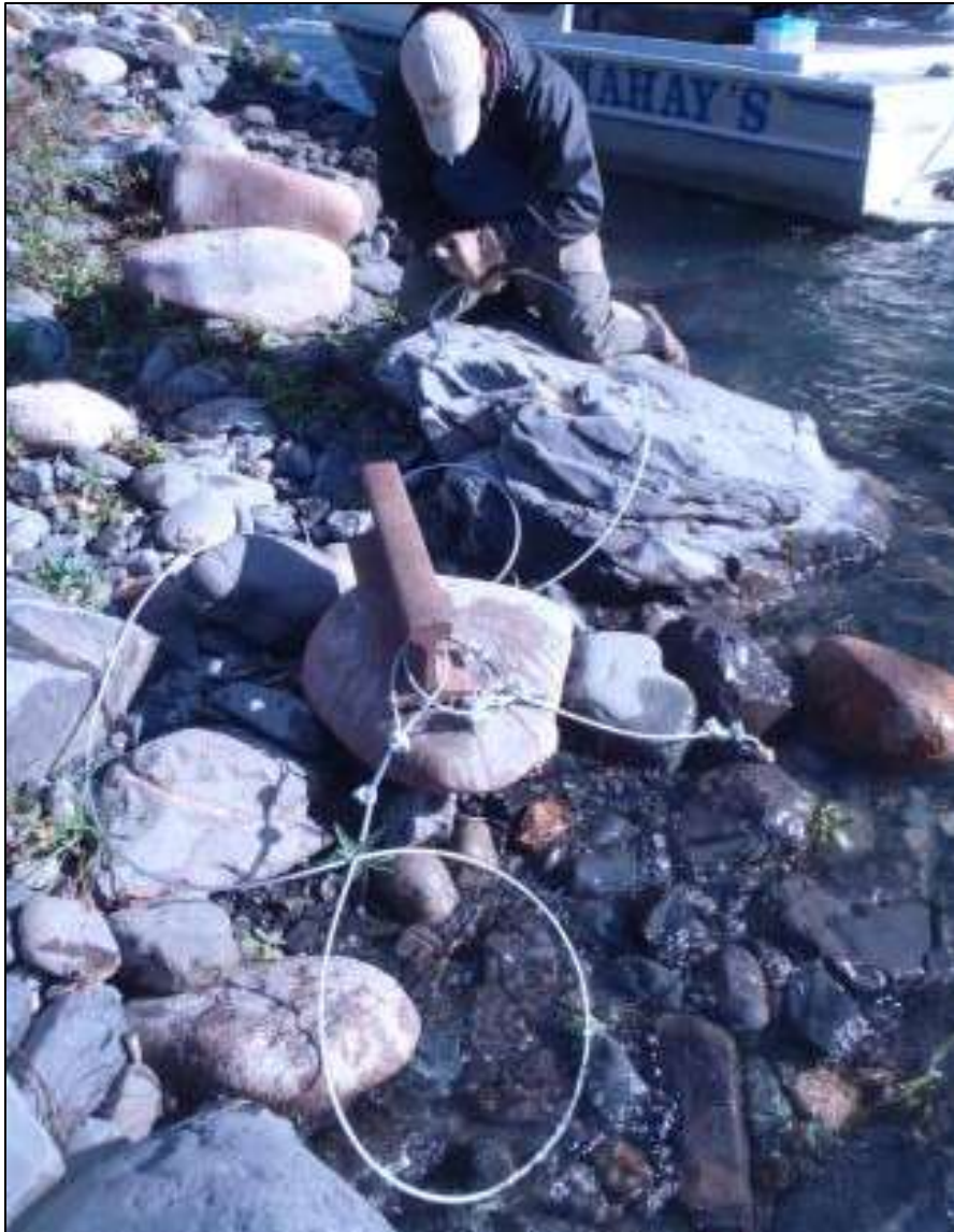
Buoy Installation at RM 148.8- Portage Creek
