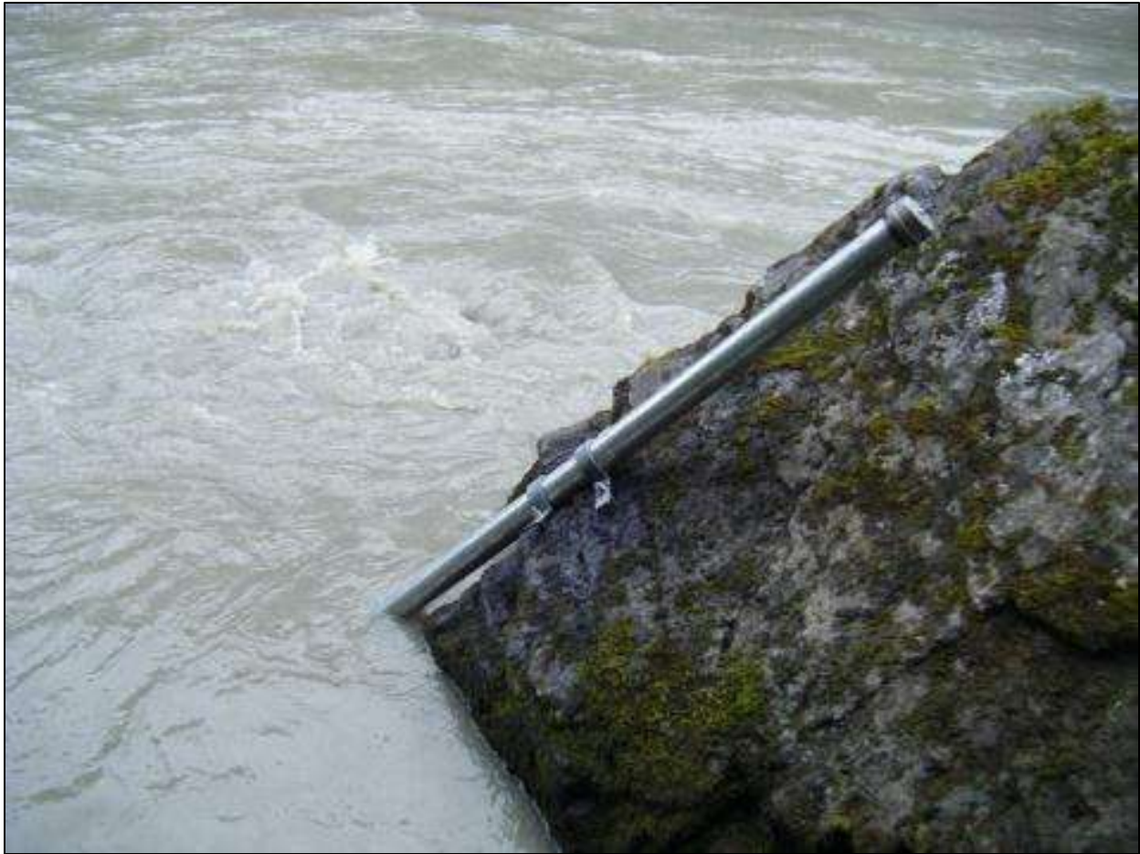
Pipe Installation at RM 148.8- Above Portage Creek
