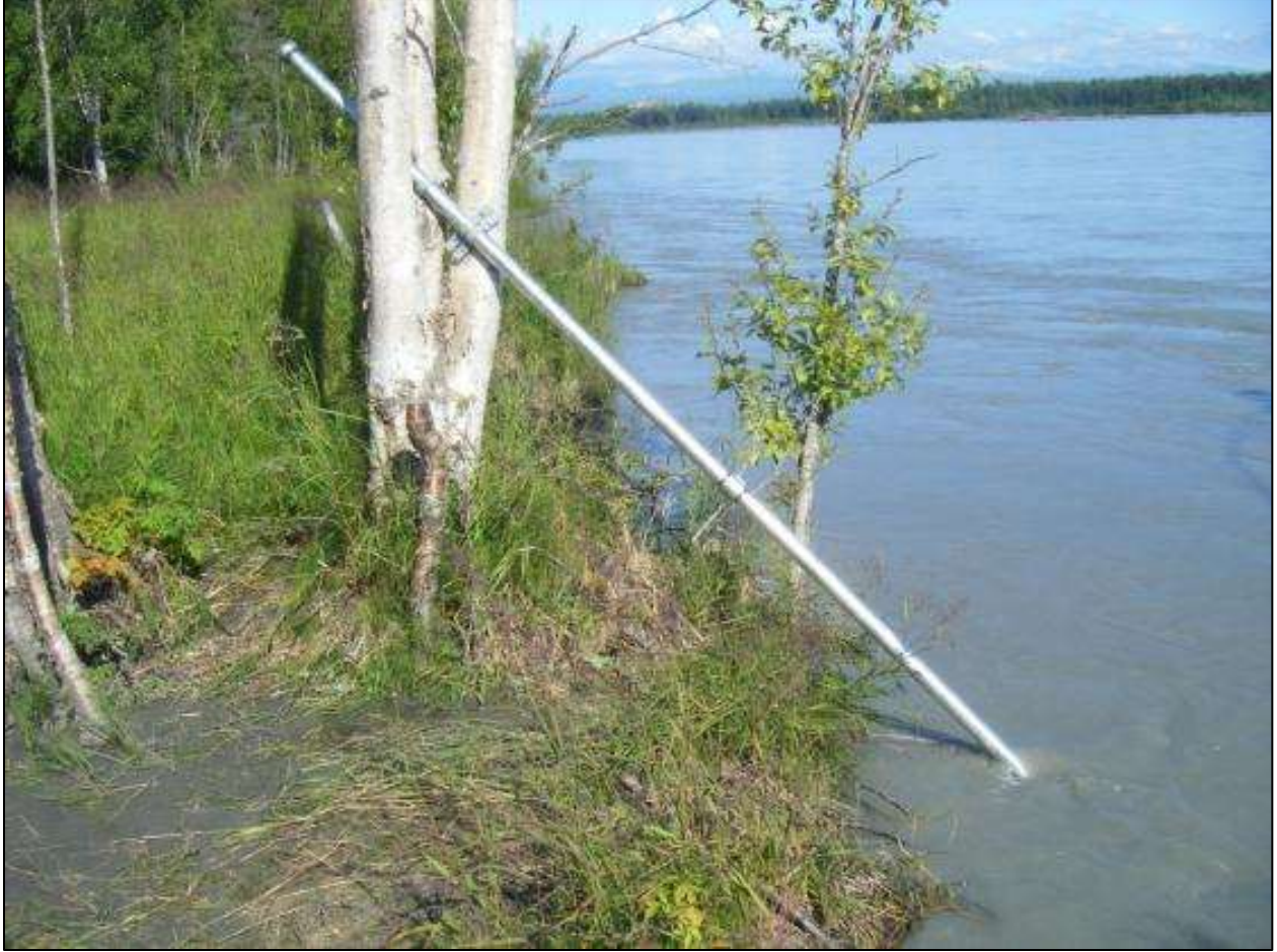
Pipe System Mounted at RM. 55.0 – Susitna
