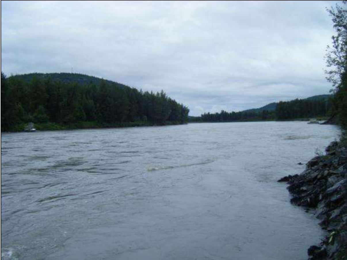
Buoy System Installed at RM 120.7- Up-River of Curry Fishwheel Camp
