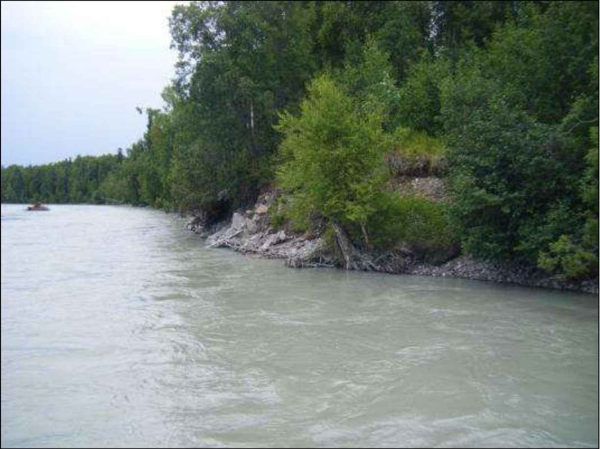
Pipe Mounted at RM 95.8 an Alternate Location for RM 97.0
