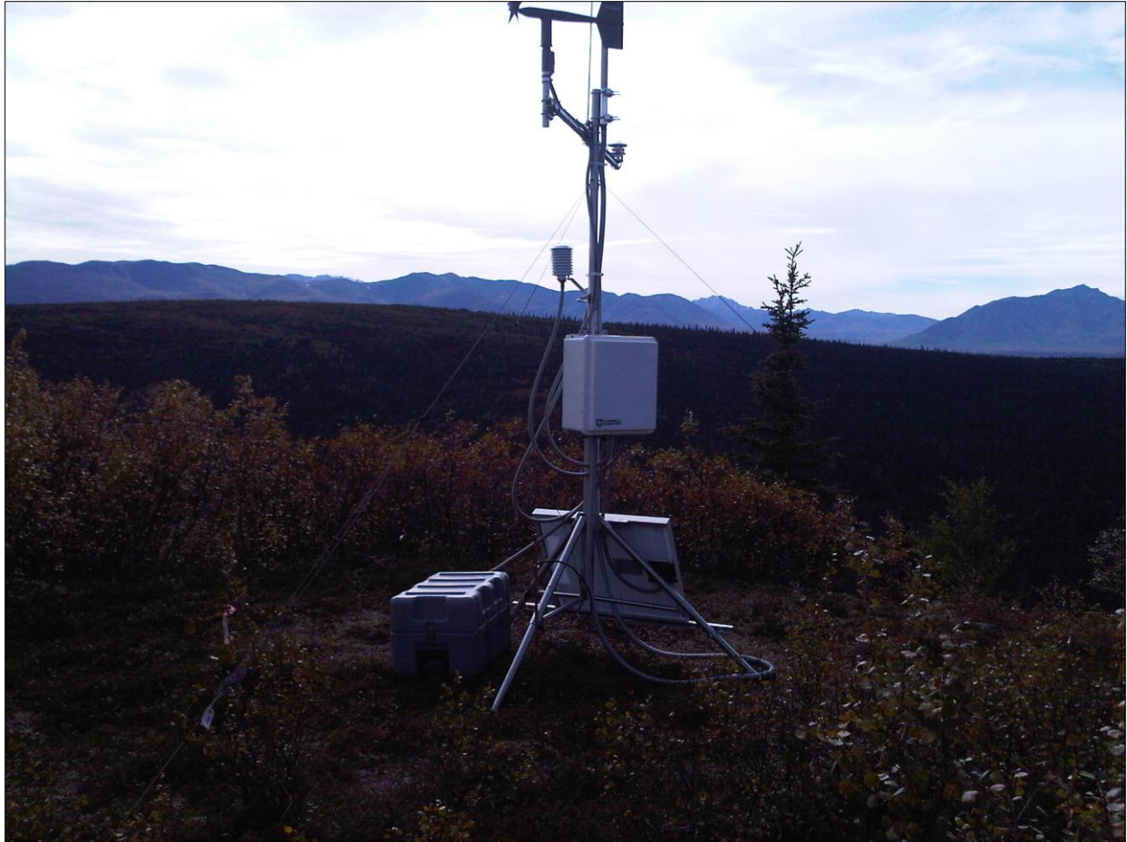
Figure 5.5-2. Example of a 10-foot (3-meter) tripod MET station installed above the proposed Watana Dam site.
