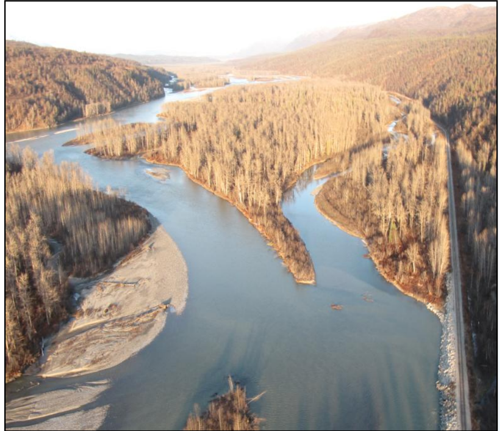
Slough 8A, Looking Upstream, 10/12/2012
