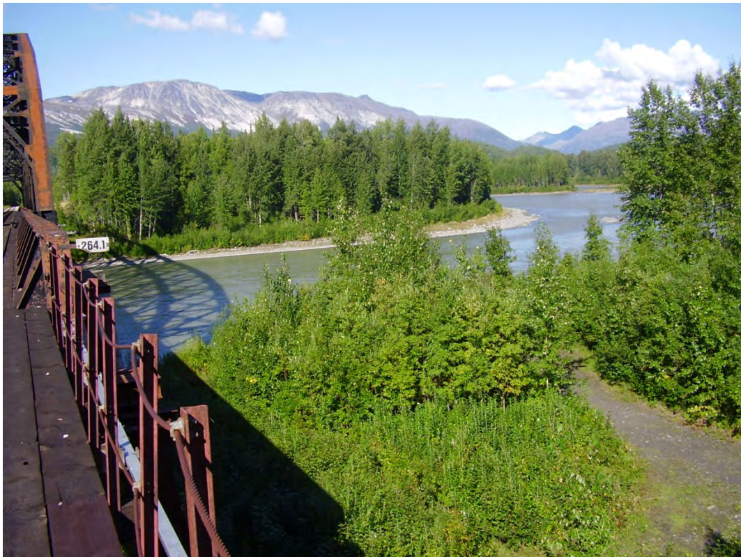
Railroad bridge crossing Susitna River near Community of Gold Creek, looking northeast
